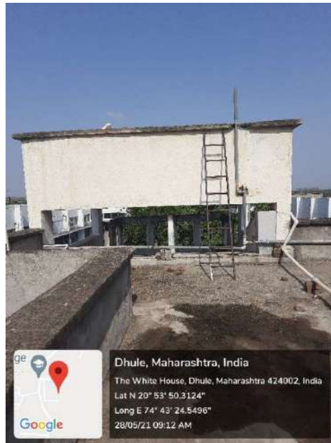
Geo Tagged Photo – Overhead tank installed on rooftop of institute
