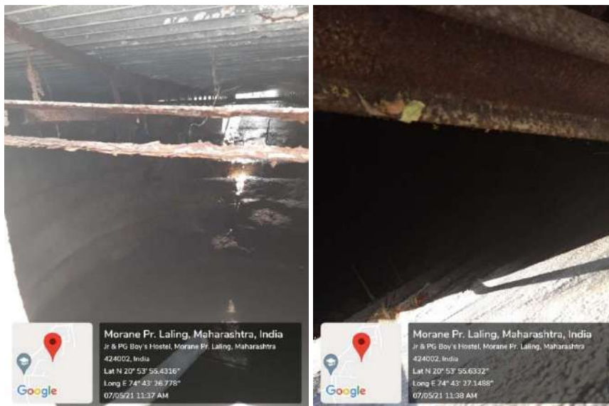
Geo tagged photo – insides of rainwater harvesting storage well
