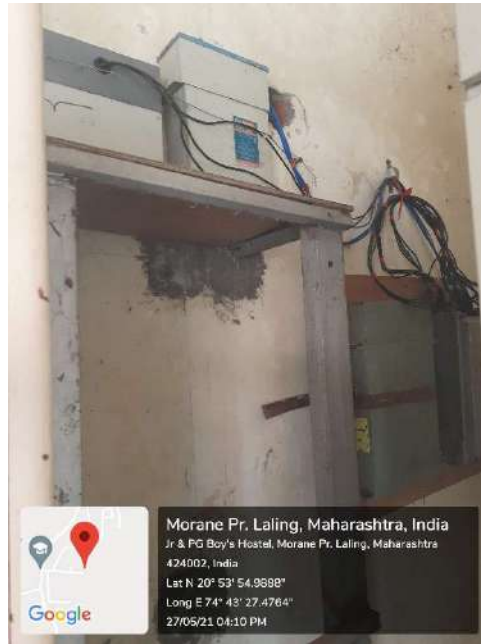
Geotagged photo – Capacitor bank installed in the campus
