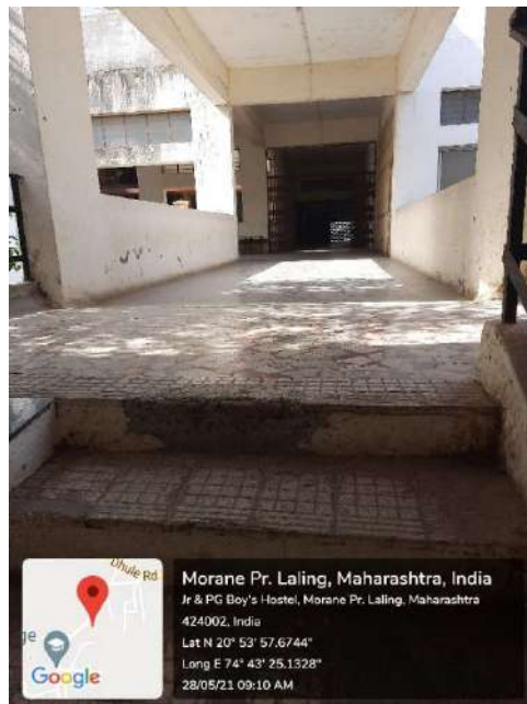
Geo tagged photo - Walkway connecting college building to hospital
