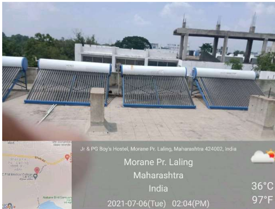
Geo Tagged Photo – Solar Water heater installed on the rooftop of Boys hostel
