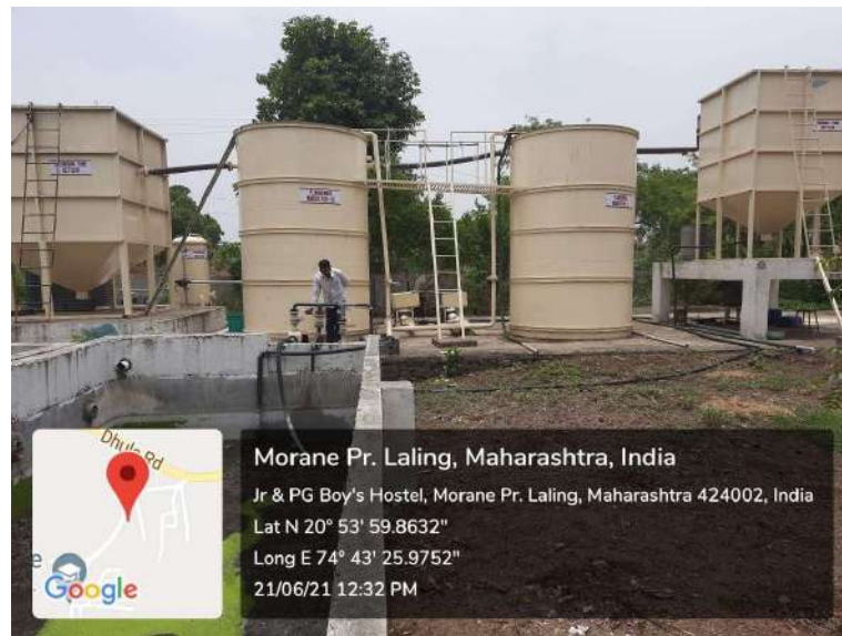
Geo tagged photo – STP installed in the campus
