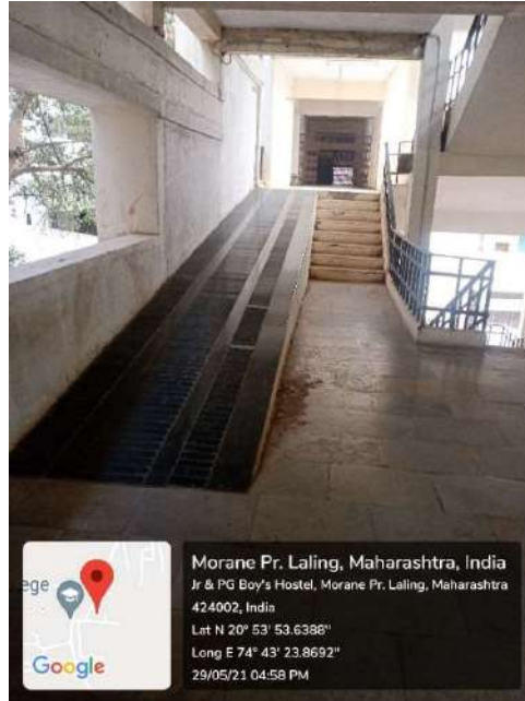
Geo tagged photo – ramp constructed in the institute for ease of movement of wheelchair
