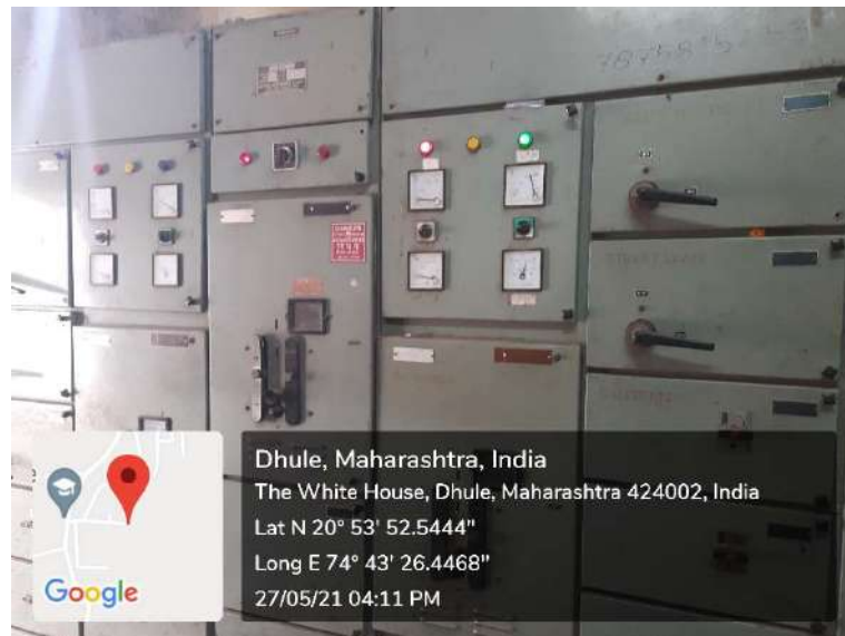
Geo tagged photo - Control panel installed for power factor indication
