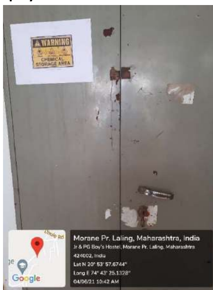
Geo tagged photo – dedicated cupboard for storage of hazardous chemicals
