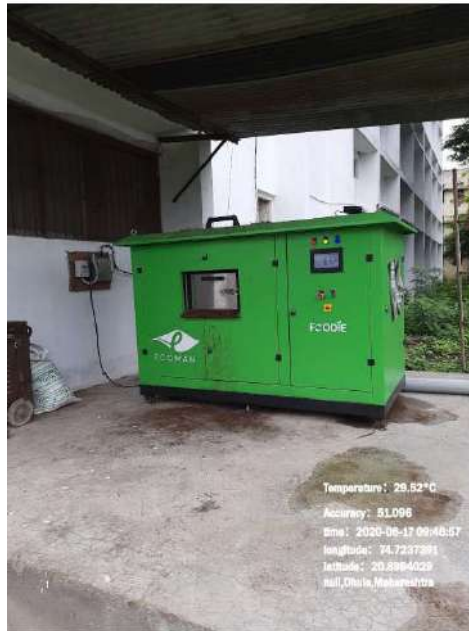
Geo tagged photo – Composter machine installed in the campus
