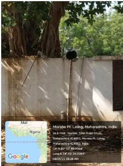
Geo tagged photo – pipeline for treated water supplied from STP to gardening
