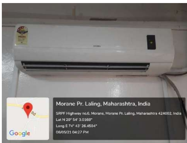
Geo Tagged Photo – Air conditioner installed in Molecular Laboratory
