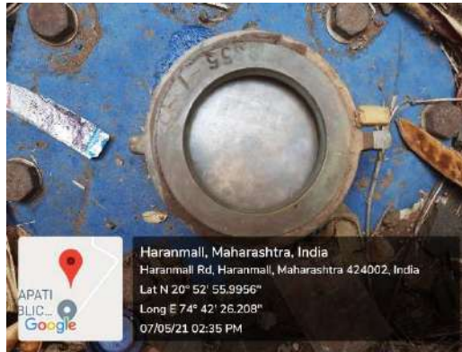
Geotagged photo – Water meter Haranmaal lake to indicate water disbursed to institute
