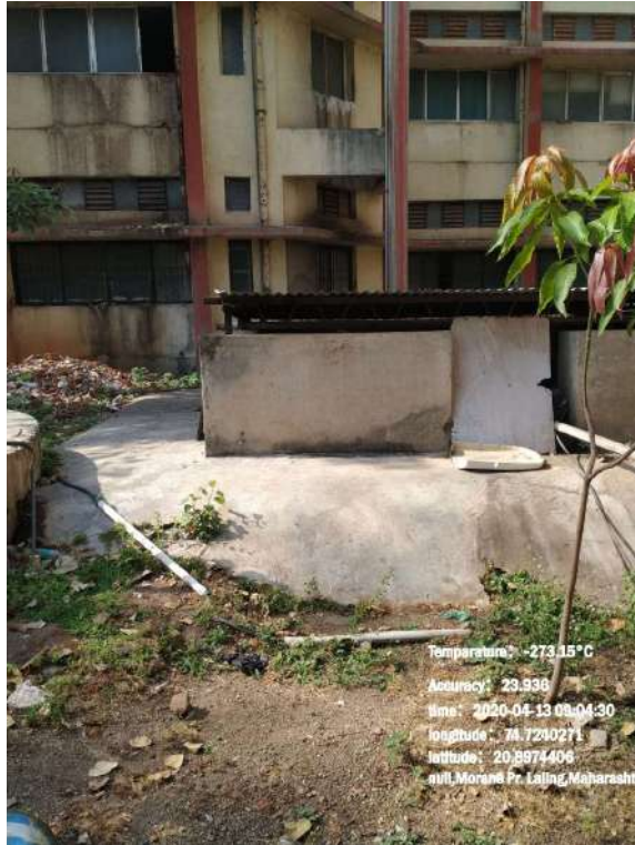
Geo tagged photo – Wells constructed in the campus.
