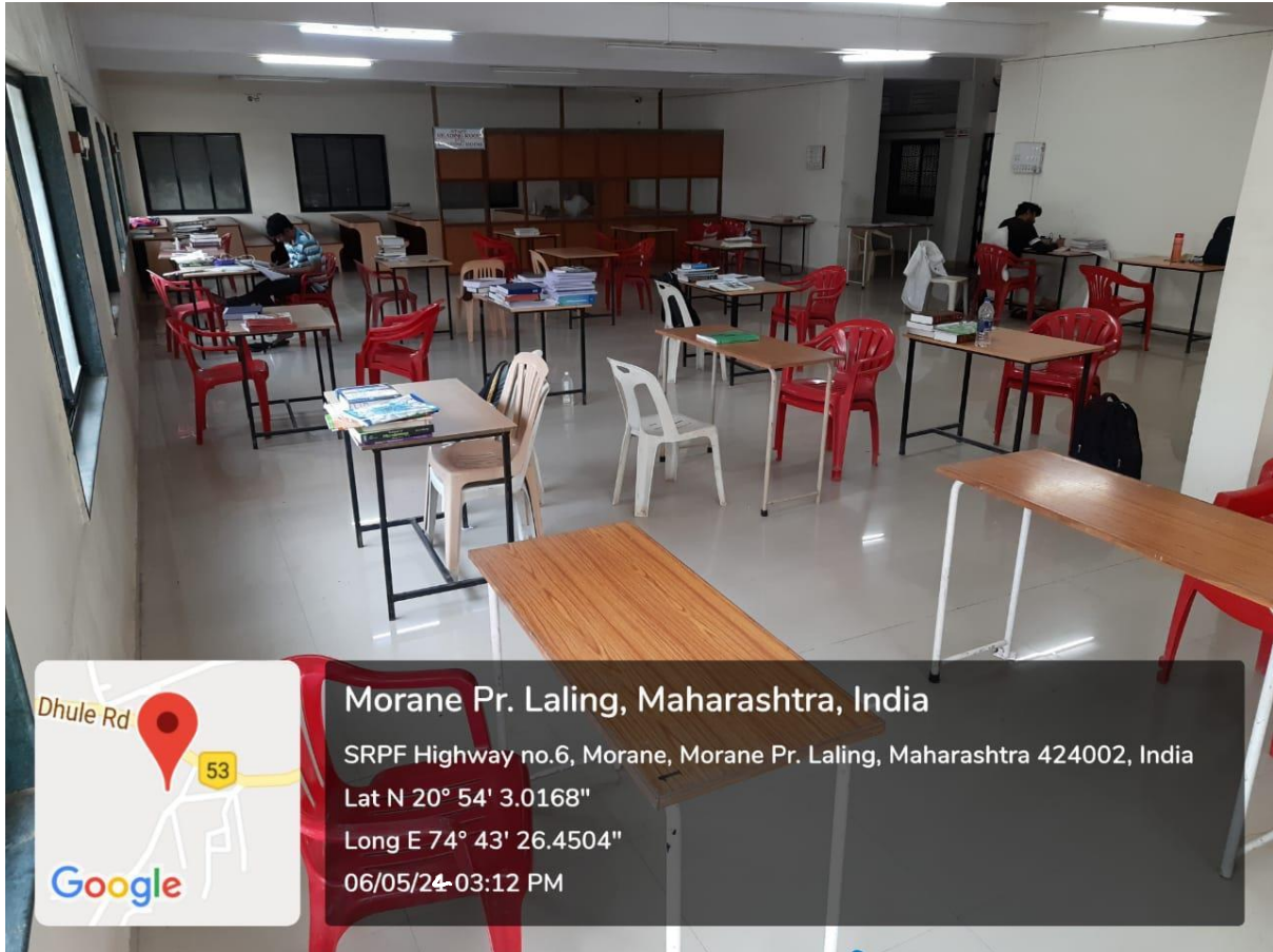
LED Lights in Library outside reading hall
