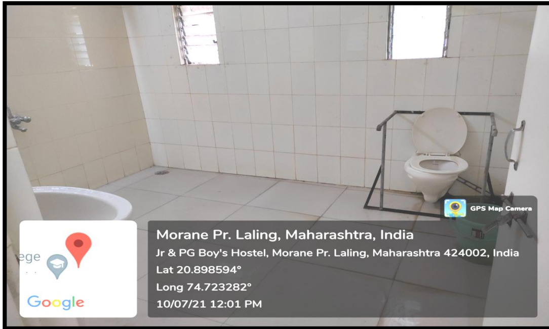
TOILET FOR DISABLED
