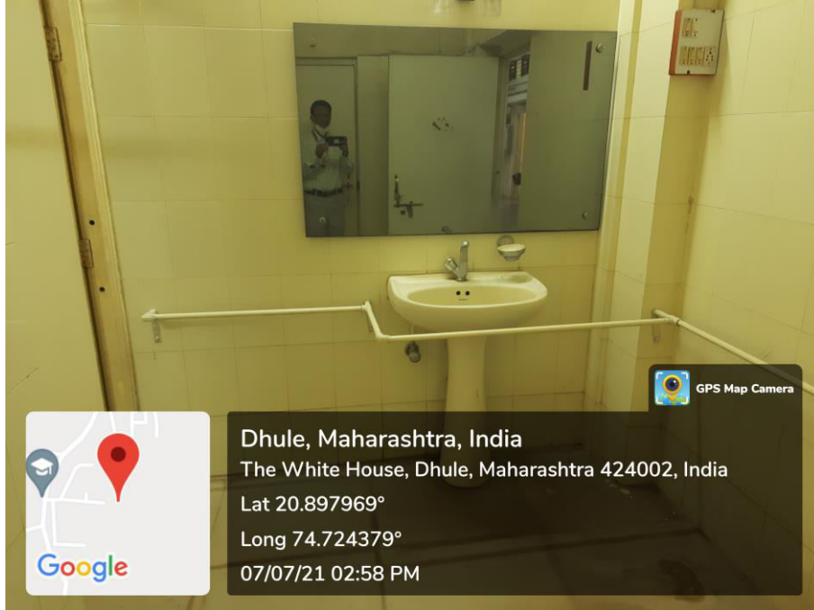
Facility for disabled in washroom
