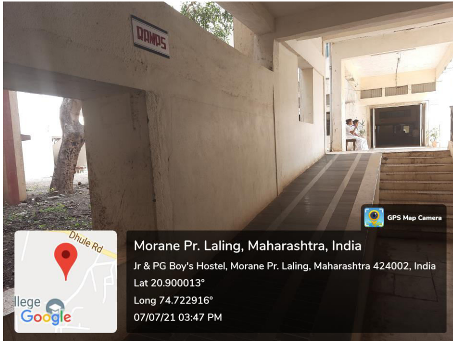
Ramp at College Building
